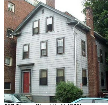
307 Thayer Street (built 1865)
