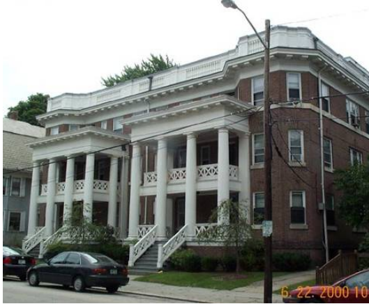
165-167 Lloyd Avenue (built 1910)
