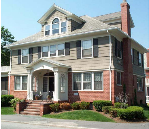
134 Hope Street (built 1910)
