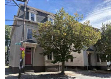
287 and 291 Brook Street
