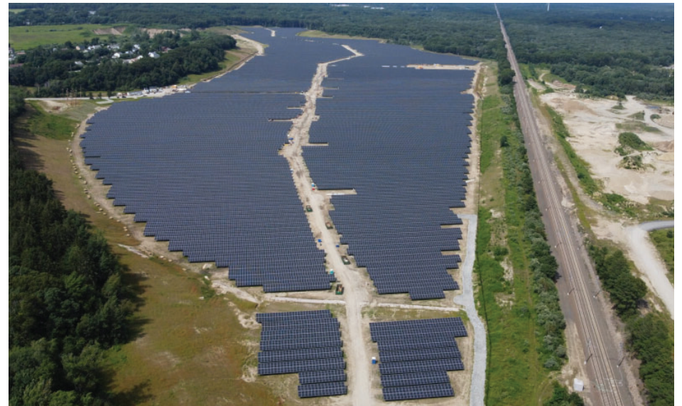
Dry Bridge Solar Field, North Kingstown, RI
