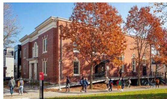
Churchill House entrance, off Angell Street
