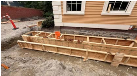
New accessible ramp
